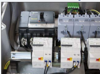
Built-in /magnetothermal circuit breakers
